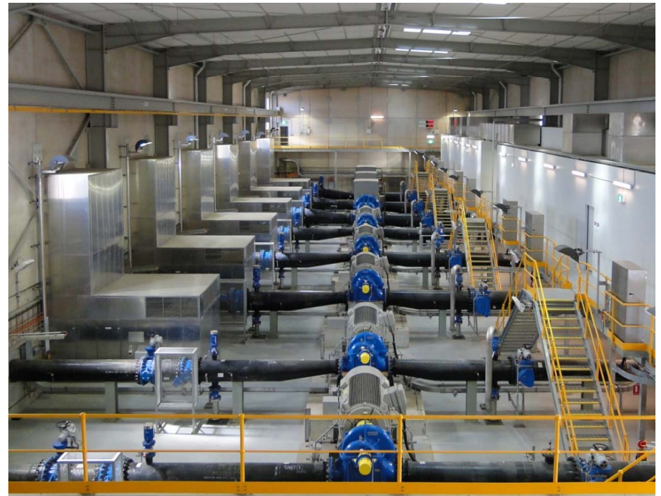
Transfer Pump Station conveying desalinated water to Happy Valley for integration into the water distribution network.
