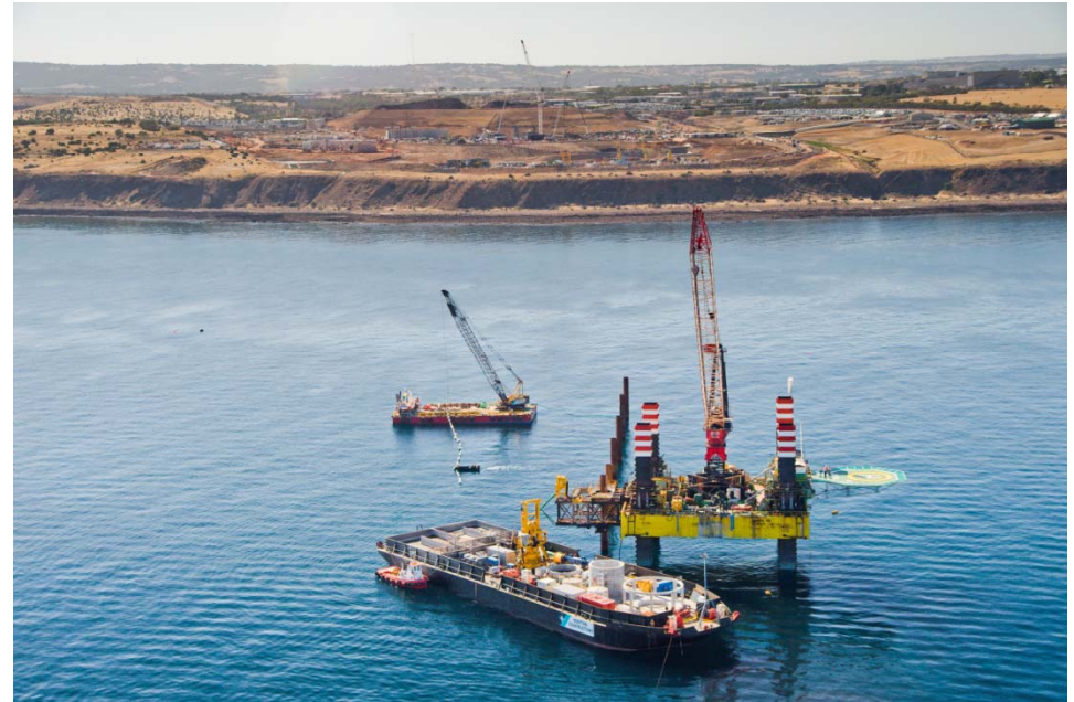
Below sea tunnelling activities supported by the Santa Fe Jack Up barge situated at Gulf St. Vincent.
