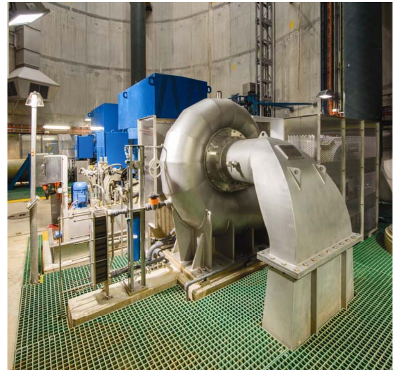
Energy recovery turbines in the outfall - generates 2.5%-3% of Plant's energy requirements at full production.
